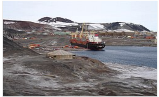
Discovery Hut (1902) at Hut Point Peninsula of Ross Island, Antarctica, one of the earliest repeatedly temporarily used dwellings on Antarctica. In the background McMurdo Station , the largest base on Antarctica today, with cargo operations of the supply ship MV American Tern of Operation Deep Freeze 2007.
