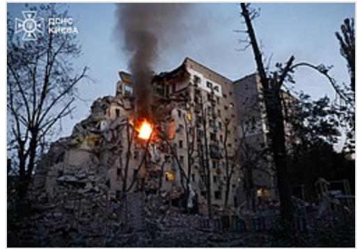
Apartment building in Kyiv after the attack
