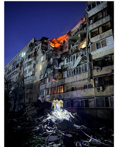
Apartment building in Kyiv after the attack
