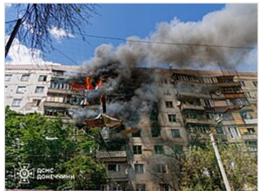
Apartment building in Kramatorsk, Donetsk Oblast, after drone strike on 16 June. Anti-drone net covering the street is seen.
