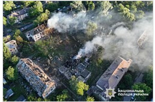
Destroyed and damaged residential buildings in Dnipro after the attack on 2 June
