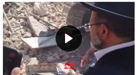
Members of the Tehran Jewish community navigating the site where the Rafi'-Nia synagogue was destroyed
