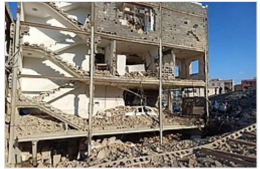
2 March: Damage to residential buildings in Sanandaj , Iranian Kurdistan
