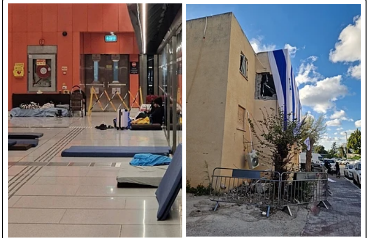
Left: Civilians sheltering in a converted light rail station in Tel Aviv on 6 March
