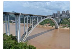
Wanzhou Yangtze River Bridge, China
