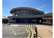
Cambridge South station eastern entrance
